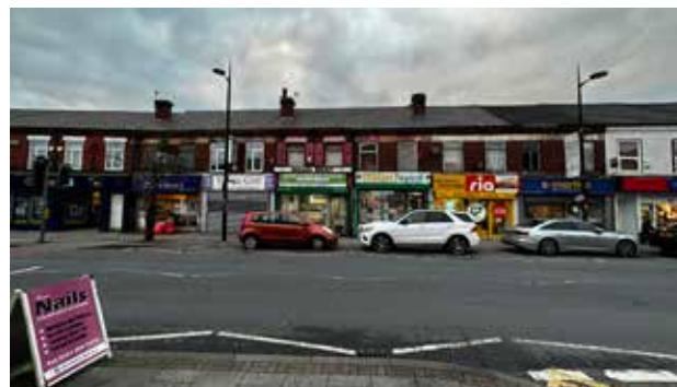
Existing shop frontages along Moston Lane
